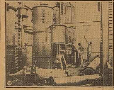
First of what is expected to become a chain of plants to produce power alcohol for automobile fuel from grain and other farm products, this factory is ready to begin production at Atchison, Kan. At left, workmen are installing the huge stills, and at right is shown the plant itself, with one of a battery of 100,000-gallon fermenting tanks. General use of such fuel is expected to relieve strain on the decreasing supply of oil in the ground and create a use for surplus farm products.
