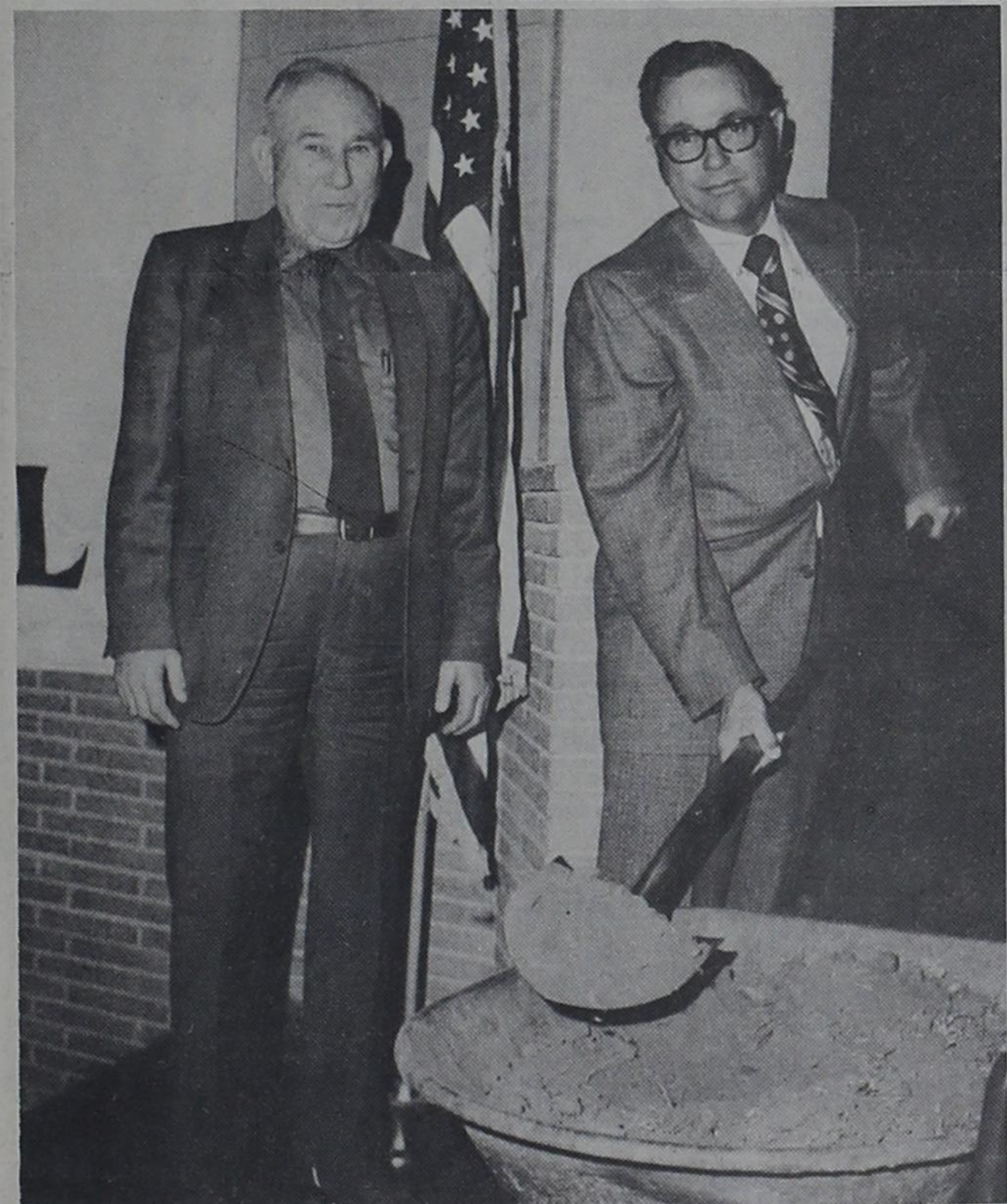
GROUND BROKEN... The symbolic "first shovel-full" of earth was turned by County Judge Archie Tarter, left, and Leon Grissom, chairman of the Soil & Water Conservation District's board of directors, at the conclusion of Tuesday's Dedication Ceremony held at the Bovina School Auditorium. The unique groundbreaking was held indoors due to cold weather.
