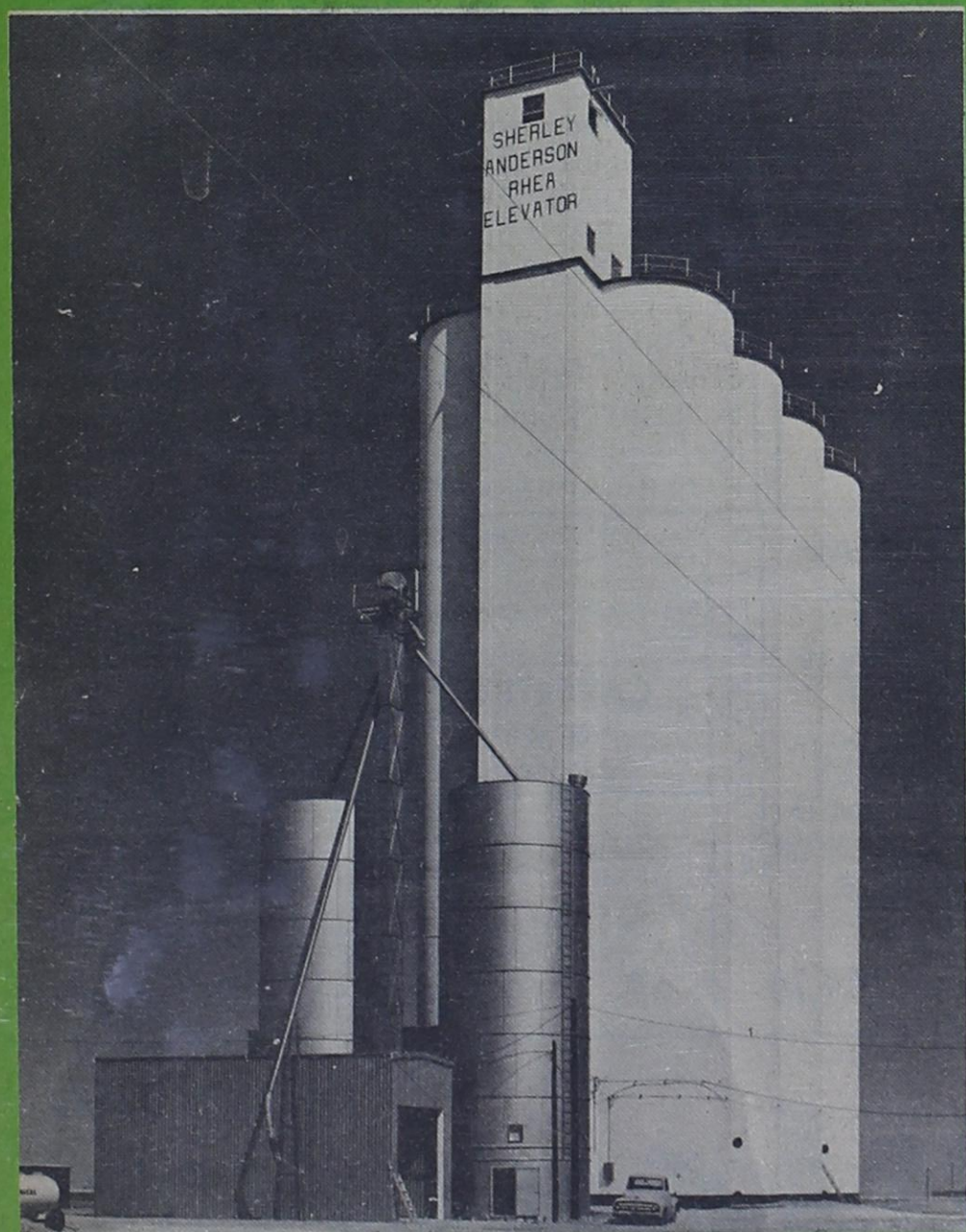
SHERLEY-ANDERSON RHEA ELEVATOR
