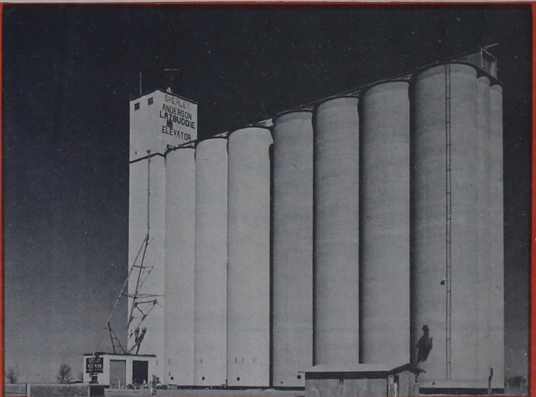
Sherley - Anderson LAZBUDDIE ELEVATOR
