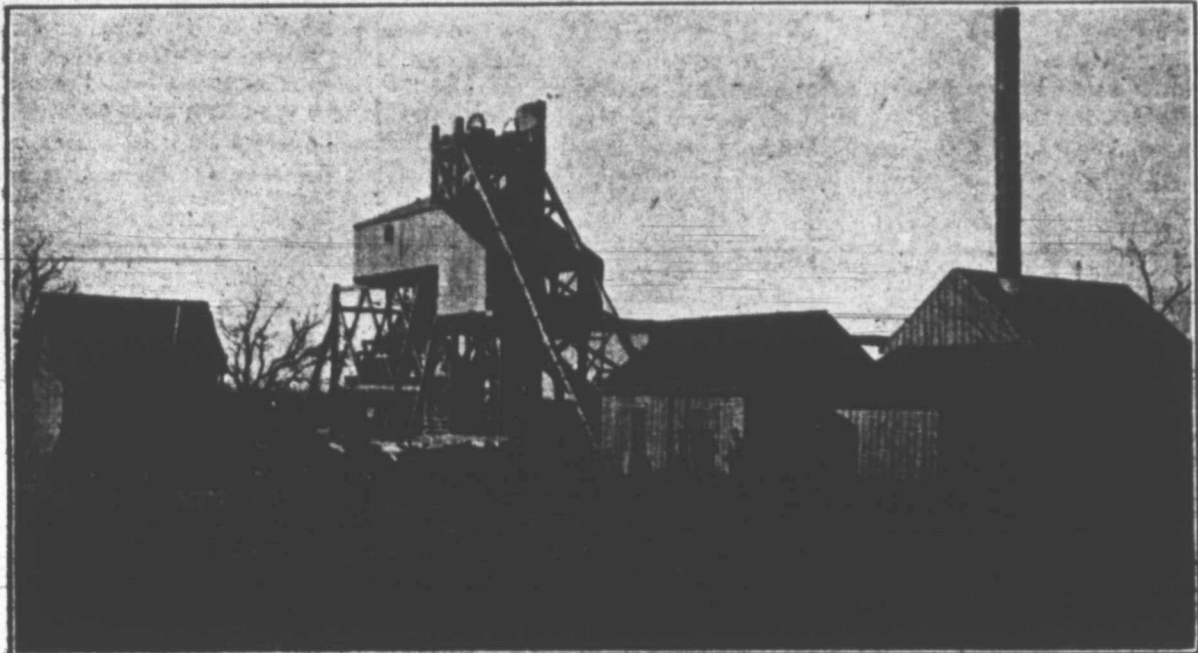
SHAFT No. 2, BELKNAP COAL CO.
