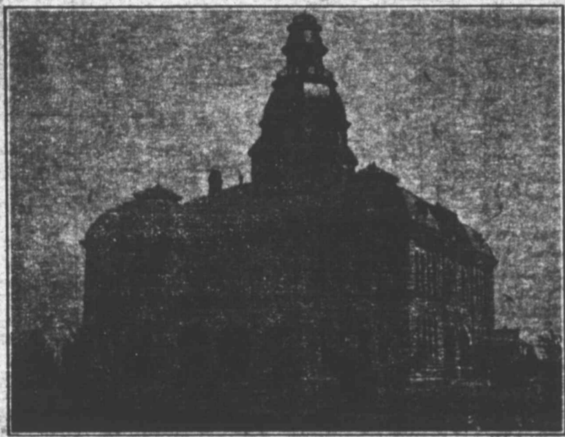
ARCHER COUNTY'S $75,000 COURT HOUSE.
