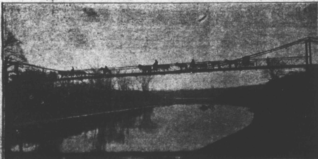
Suspension Bridge Built By Residents of the Byers Country, Without Assistance of the County Commissioners.
