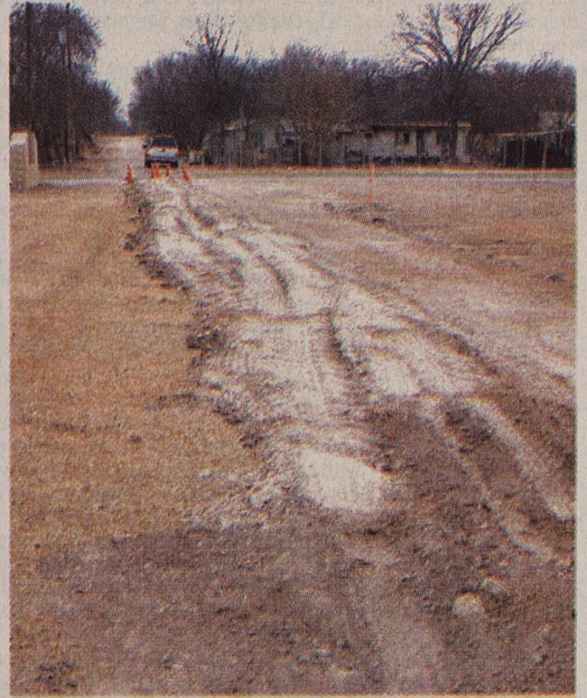
Brackett News Weekly Photo By Leigh Jenkins - From left: Damage to the walls in the Fellowship Hall at Frontier Baptist Church. Frontier Baptist Church Pastor Ned Sitzes explains the flooding and repair process; and the covered trench that encases a new PVC pipe.
