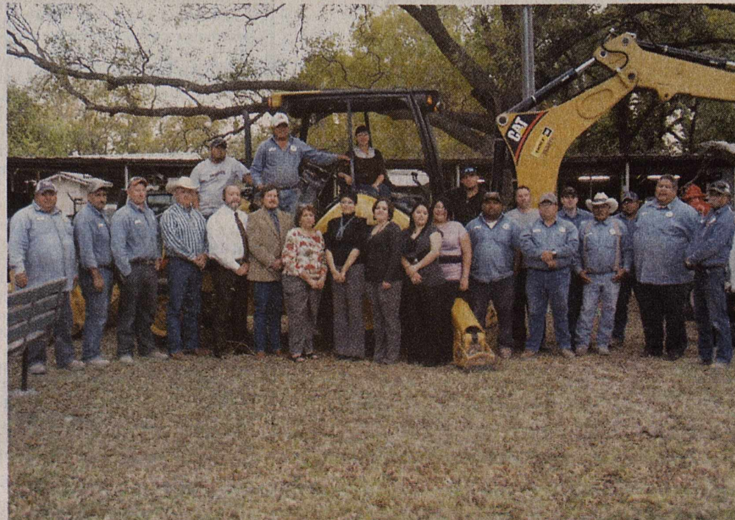
Brackett News Photo By Leigh Jenkins - City Employees gather to celebrate the beginning of the water line repair project that will be funded by a grant recently received by the city.
