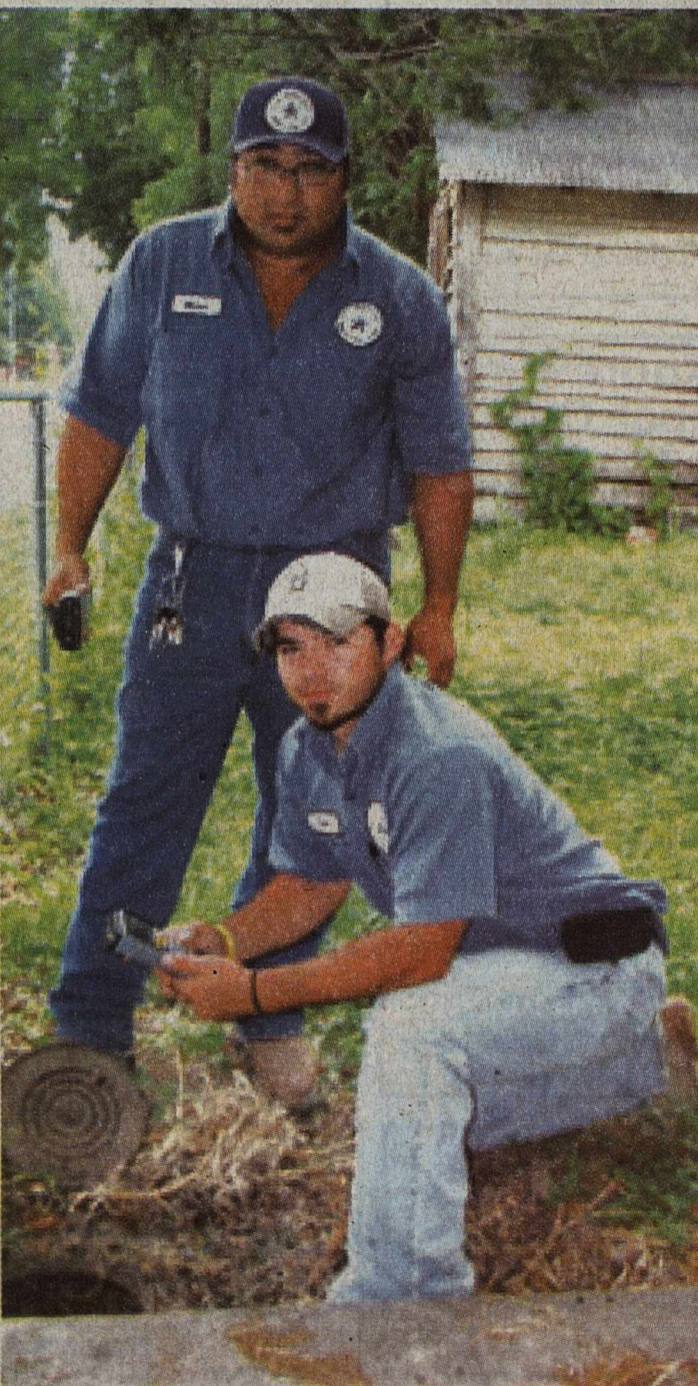
Brackett News Photo By Leigh Volcsko - City of Brackettville goes digital. City maintenance employees Marc Rodriguez and Clint Conrad test the new digital meter reading devices. The city will begin using the new technology this month.
