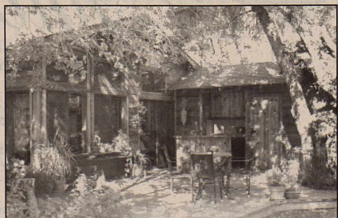
The Simmons home, left, served as the blacksmith shop to the Fort's Cavalrymen. Rebuilt in 1931, the Administrative and Member Services Building, right, served as a kitchen originally. Sunday's event is from 2 to 5 p.m.
