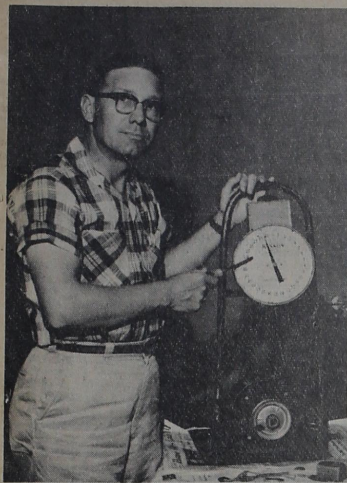
Roy Crawford, Bovina Vocational Agricultural Teacher, checks starting characteristics of electric motor at Motor Lesson Workshop sponsored by Southwestern Public Service Company in Amarillo last Tuesday and Wednesday. School was put on for Area I teachers.
