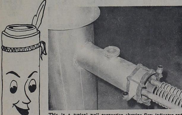
This is a typical well connection showing flow indicator and cooling coils installed by Comanche Irrigation Supply Company.
