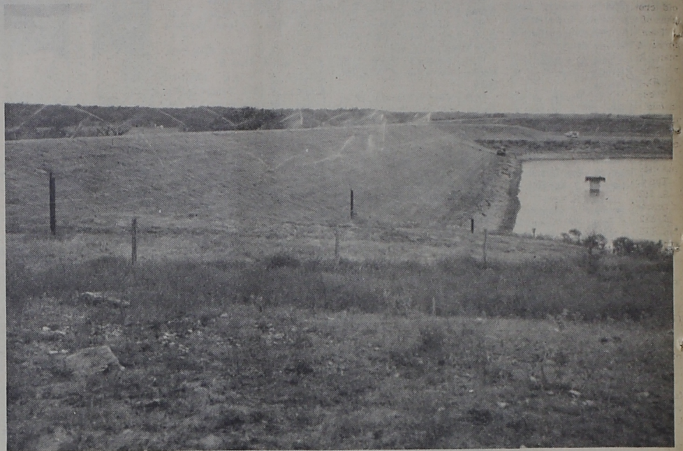
Irrigating Bermuda grass on a floodwater retarding structure by use of a sprinkler system pumping water from the lake area. This is the type of structures that are proposed for the Running Water Draw project. Note the draw-down tube to maintain a
