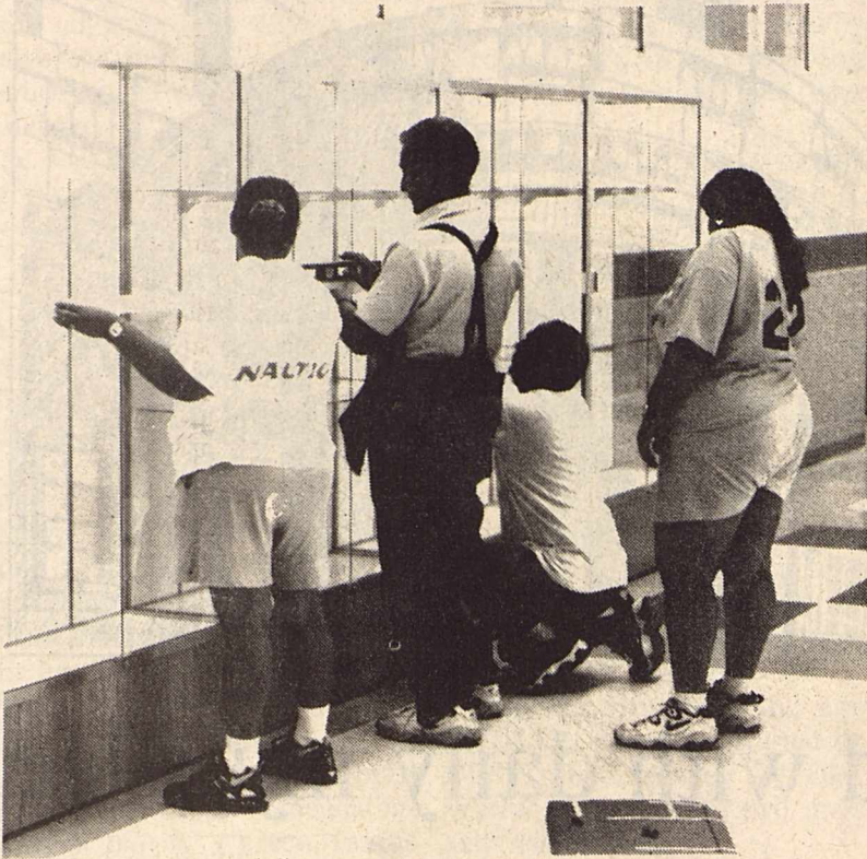
Pictured above are Brackett ISD Custodial Workers, (L to R) Eresmi Aguirre, Ruben Buantello, Tommy Castillo, and Laura Gomez. They were installing the trophy case this past Friday in the new high school building.
