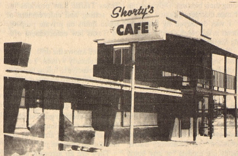
The Full Circle Cafe has had to close its doors because of a kitchen fire last week. Brackett News Photo by J.J. Guidry
