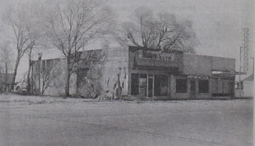
SEEN BETTER DAYS--- These old buildings located on the west end of Bovina's Main Street have been condemned and are being torn down for safety reasons.
