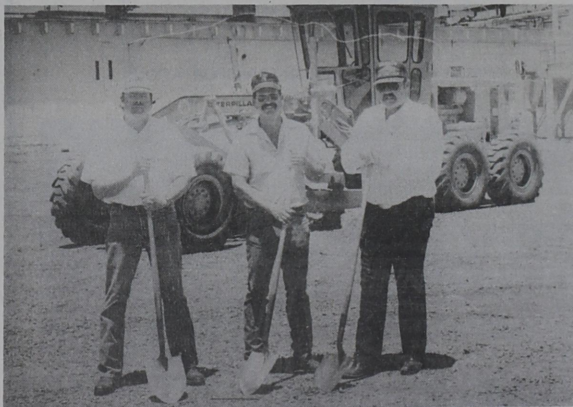
RECENT EXPANSION.... A ground-breaking was held at Friona's Excel plant in June of 1991 for the $11 million expansion project at the plant. From the left are Guy Hunter, project manager; Randy Highsmith, construction engineer; and Jacky Messer, contractor.
