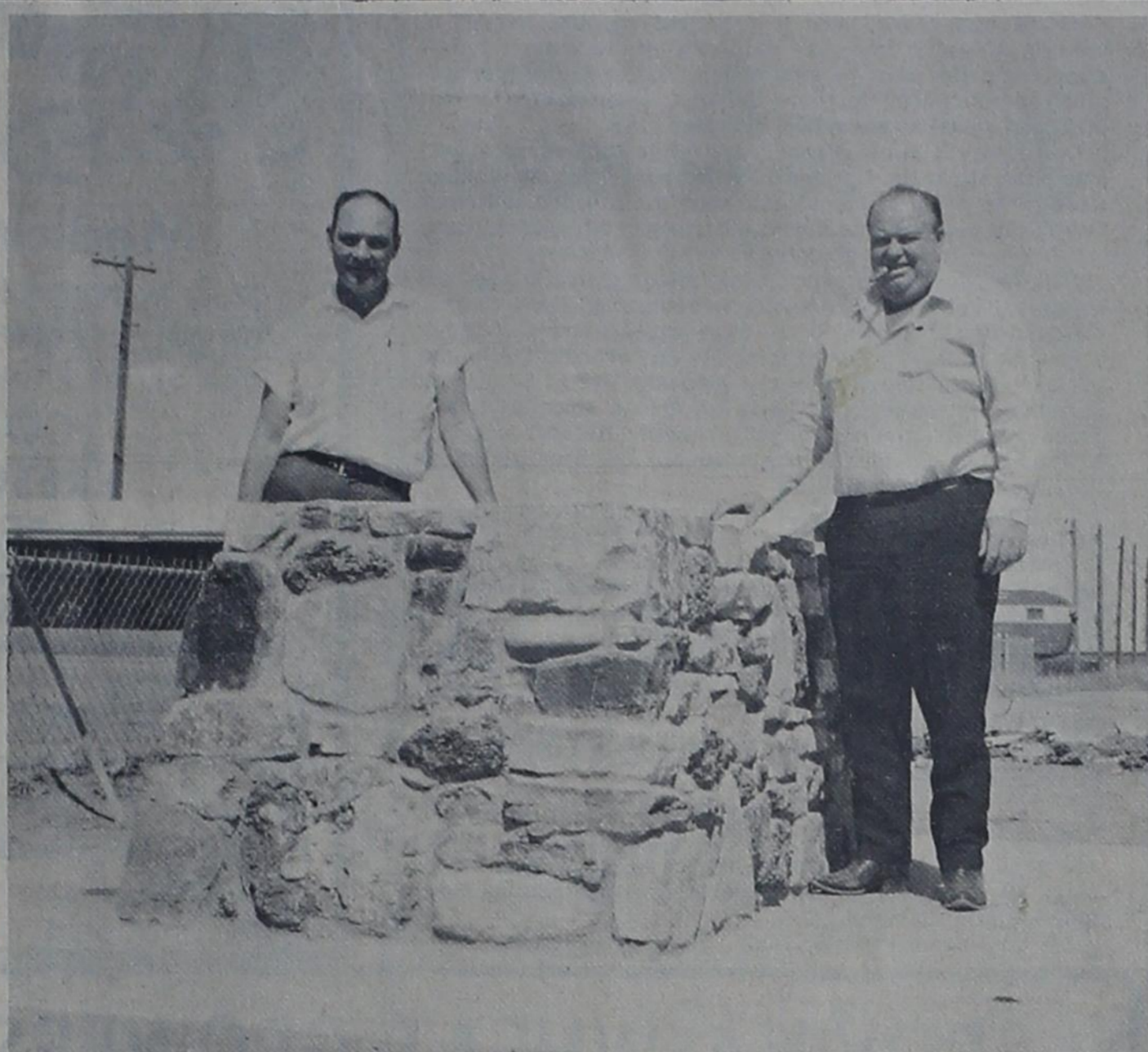
BULL PLATFORM -- Mutt Graham and Nick Trienen admire the rock platform erected this week by Bovina Roping Club for the bull statue now being sculptured in pre-colored concrete. Location of the platform is on city property on Highway 60 between Sands Motel and Bovina Restaurant. The statue is expected to be completed in July and placed on the platform by Bull Town Days.
