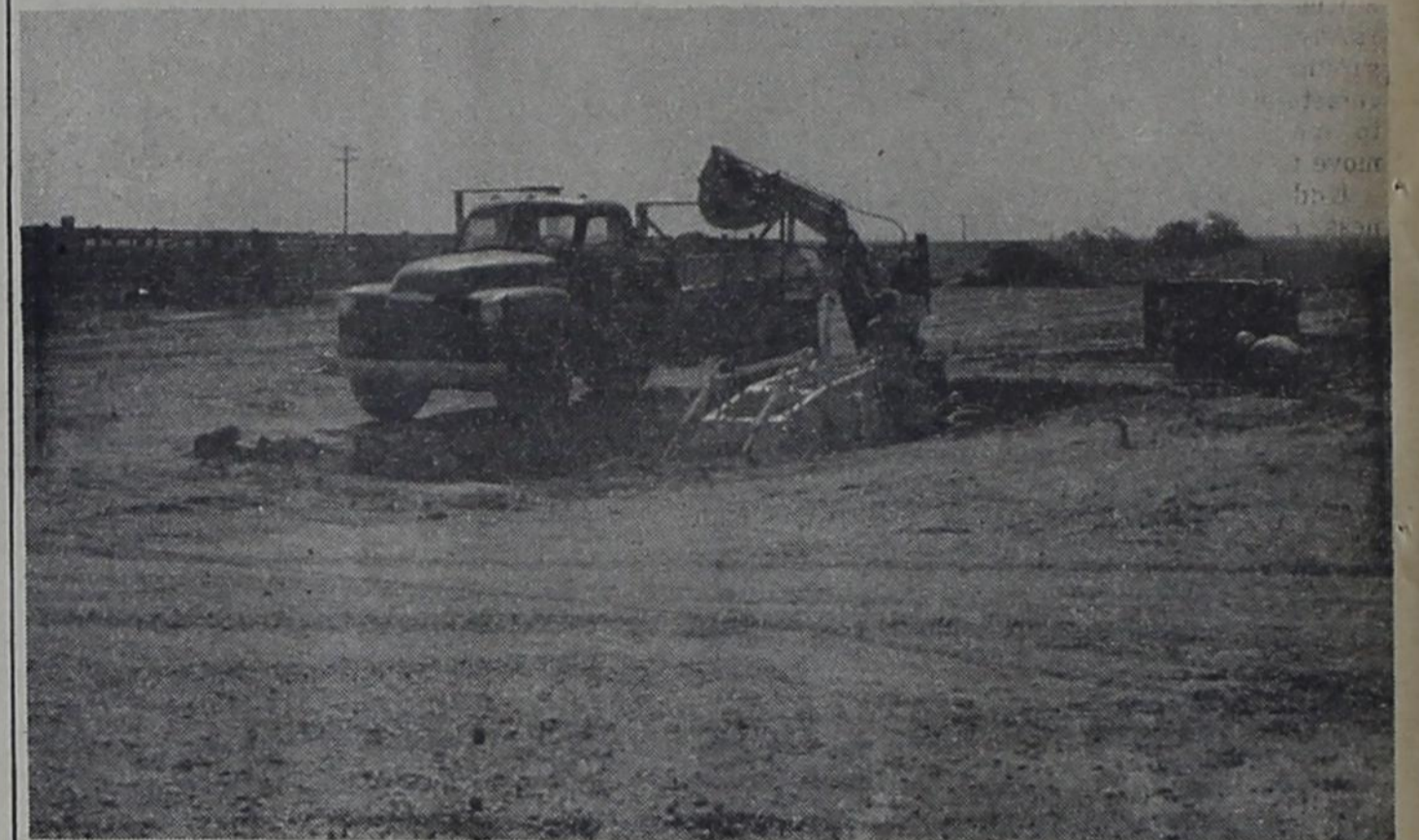
WHEAT GROWERS EXPANSION BEGINS--Men and machines began groundwork for an addition to Bovina Wheat Growers Elevator that will triple its storage capacity. The machine in the hole is preparing a place for an additional truck dump.
