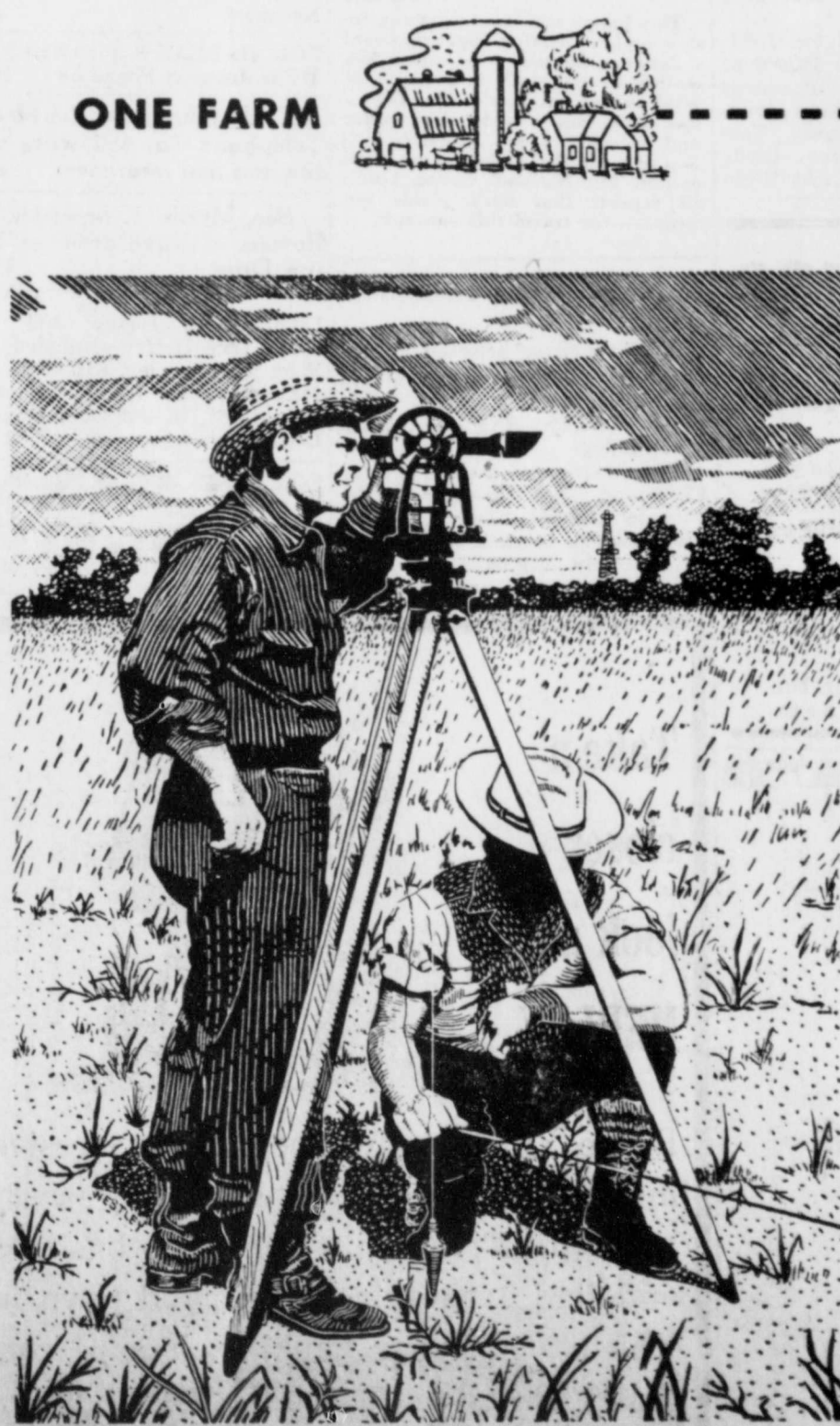
United Gas survey crew lays out a right-of-way for a new United Gas pipe line.
