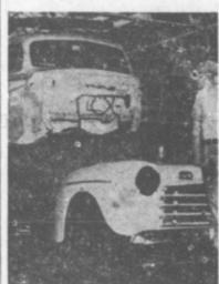
With industry given the go-ahead signal for civilian production, manufacturers strove for speedy output for the pent-up postwar market. Here, body is being slung on chassis of one of the first cars to roll off of postwar production line.
