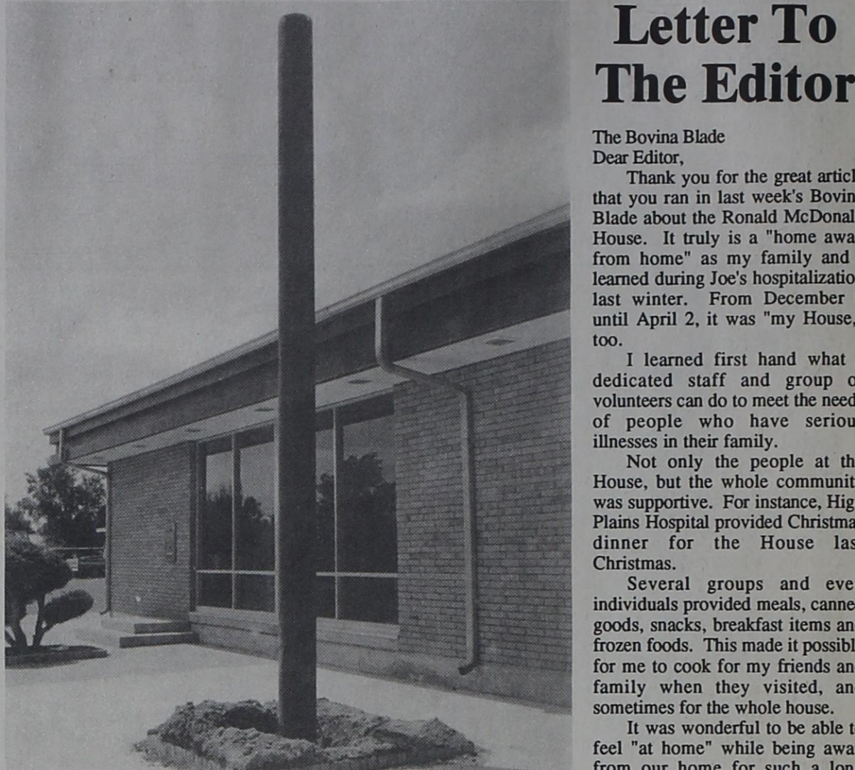
JUST STANDING AROUND....It's just a pole now, but soon it will grow and blossom into a time, temperature and message center at First Bank-Bovina. Construction is expected to be completed within the next few weeks.
