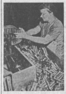
woman's touch is used at the Frankford arsenal, Philadelphia, Pa., to feed these 50-calibre cartridge cases into the machine that tapers them. These cartridges are used in anti-tank guns.
