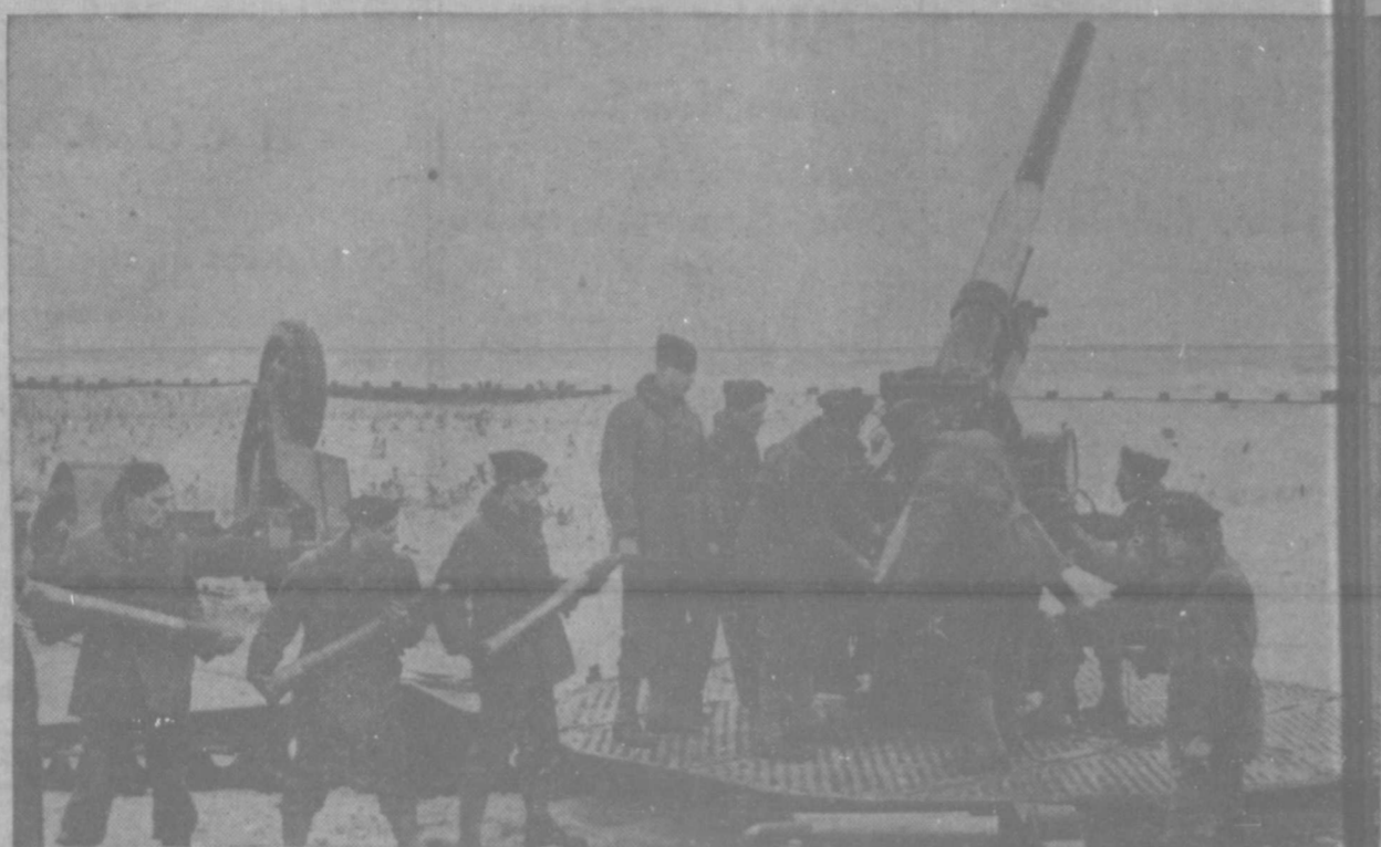
National Guardsmen of Battery D, 212th coast artillery unit, only National Guard anti-aircraft unit in New York state, load a three-inch, super-powered gun, one of 325 ordered by the government. The new weapons, which would defend New York city in case of air attack, have a three-inch bore, fire a 28-pound projectile containing 253 one-half-inch lead pellets, and can fire 30 shells a minute. Guns were tested at Fort Tilden, Rockaway beach, New York city. It was the first time since 1917 that a N. Y. National Guard regiment held winter maneuvers.
