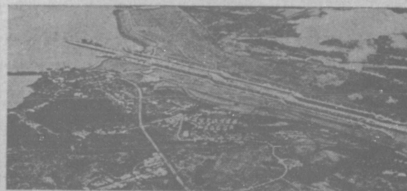
Canal locks, at the western end of Panama canal.
