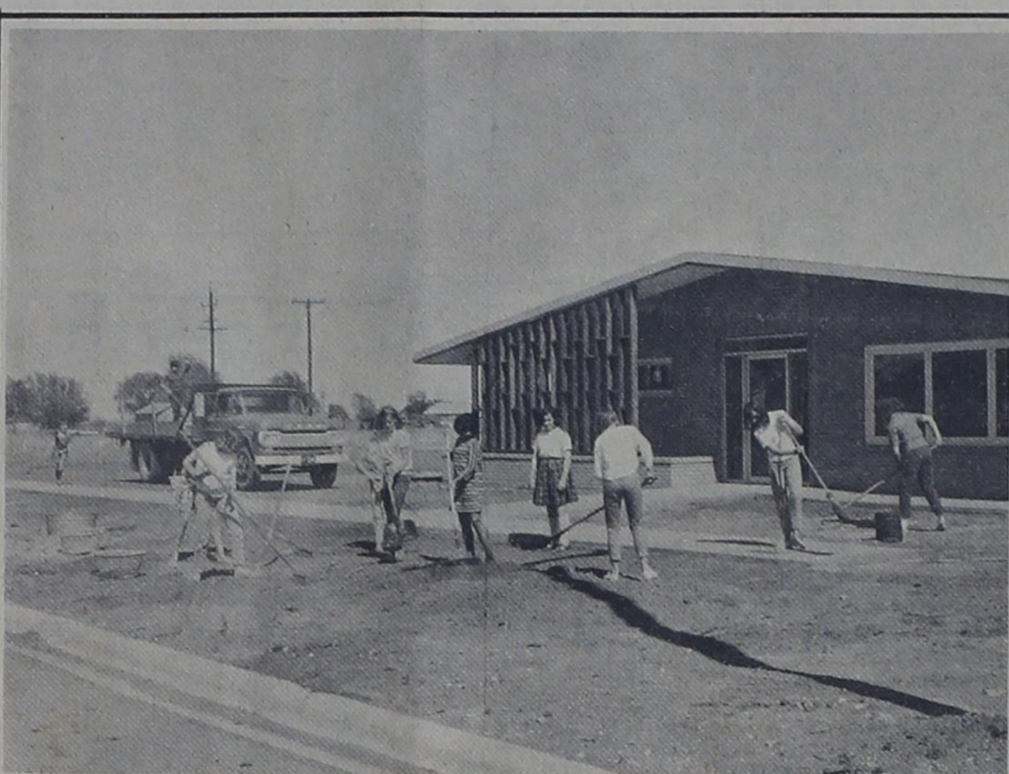
CLEAN UP -- Girl Scout Troop No. 35 became a work unit Monday afternoon when the members spent their meeting time cleaning the yard of the new Bovina Medical Clinic. The building, constructed by Sherrill Lumber Company, is scheduled to be inspected by the building committee this week.
