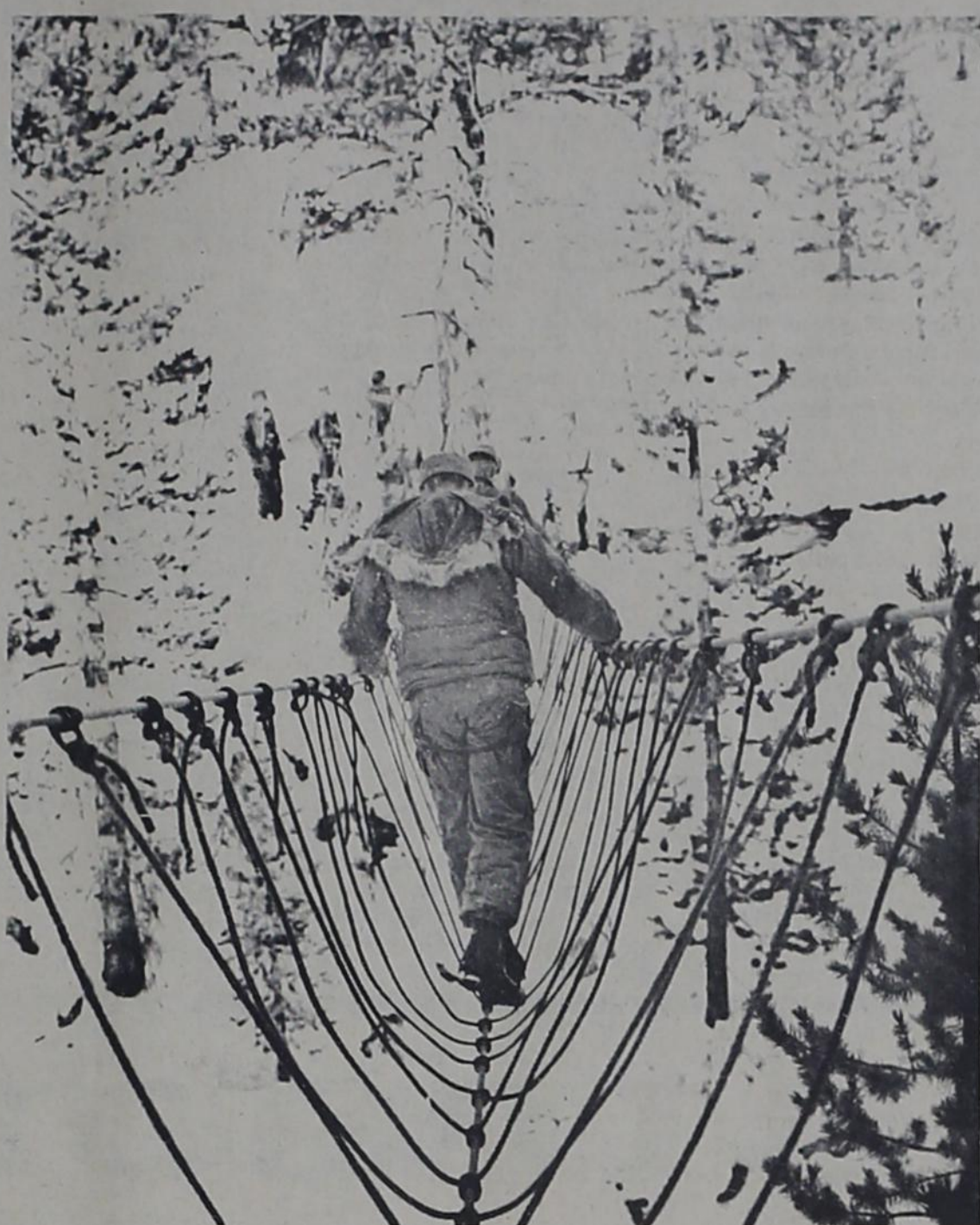
Rope bridges provide Marines with safe passage over streams and gulleys. These men are trained to improvise whenever ready made or natural facilities are not available.
