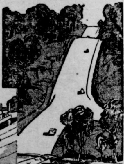
Very seldom are hills as steep as this. The average grade of highway hills is seven per cent. This hill is 25 per cent and a car must be good to make it.
