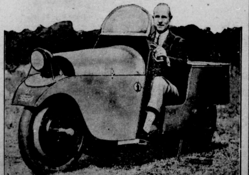
Mr. A. V. Roe, the famous airplane designer and pilot, seated in his unique motor cycle which has all the comforts of an automobile. It has a three-horse-power Villiers engine, is shaft driven and can attain a speed of 60 miles per hour. The steering is similar to that of an automobile and the driver sits on an upholstered seat and back.
