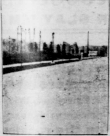
Experimental Concrete Road, Chevy Chase, Md., After Nearly Two Years' Service.
