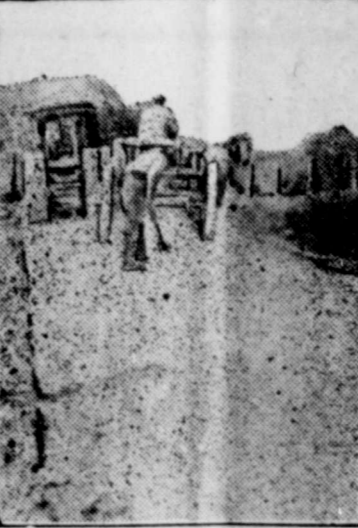
Building an Up-to-Date Highway.
