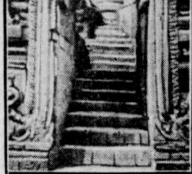
ONE OF THE STEPPED ARCHES.
