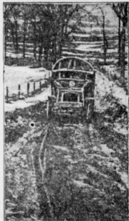
Road Cleared for Passage of Motor-trucks.
