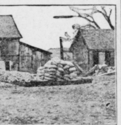
Concreting the Barnyard of C. W. Lau Farm.
