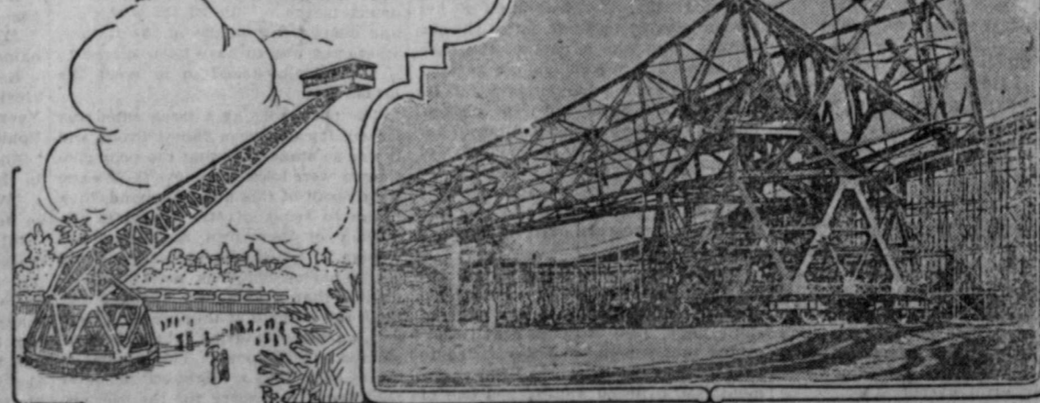
THE GIANT FRAME OF THE AEROSCOPE AS IT APPEARED UNDER CONSTRUCTION
