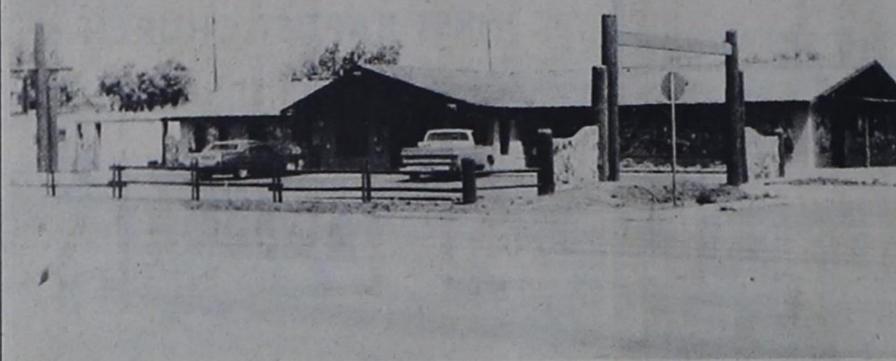
NEW FACILITY ...Pioneer Cattle Order Buyers has recently moved into their new building on Highway 60 in Friona. The company is hosting open house activities for Saturday and Sunday, to which the public is invited.
