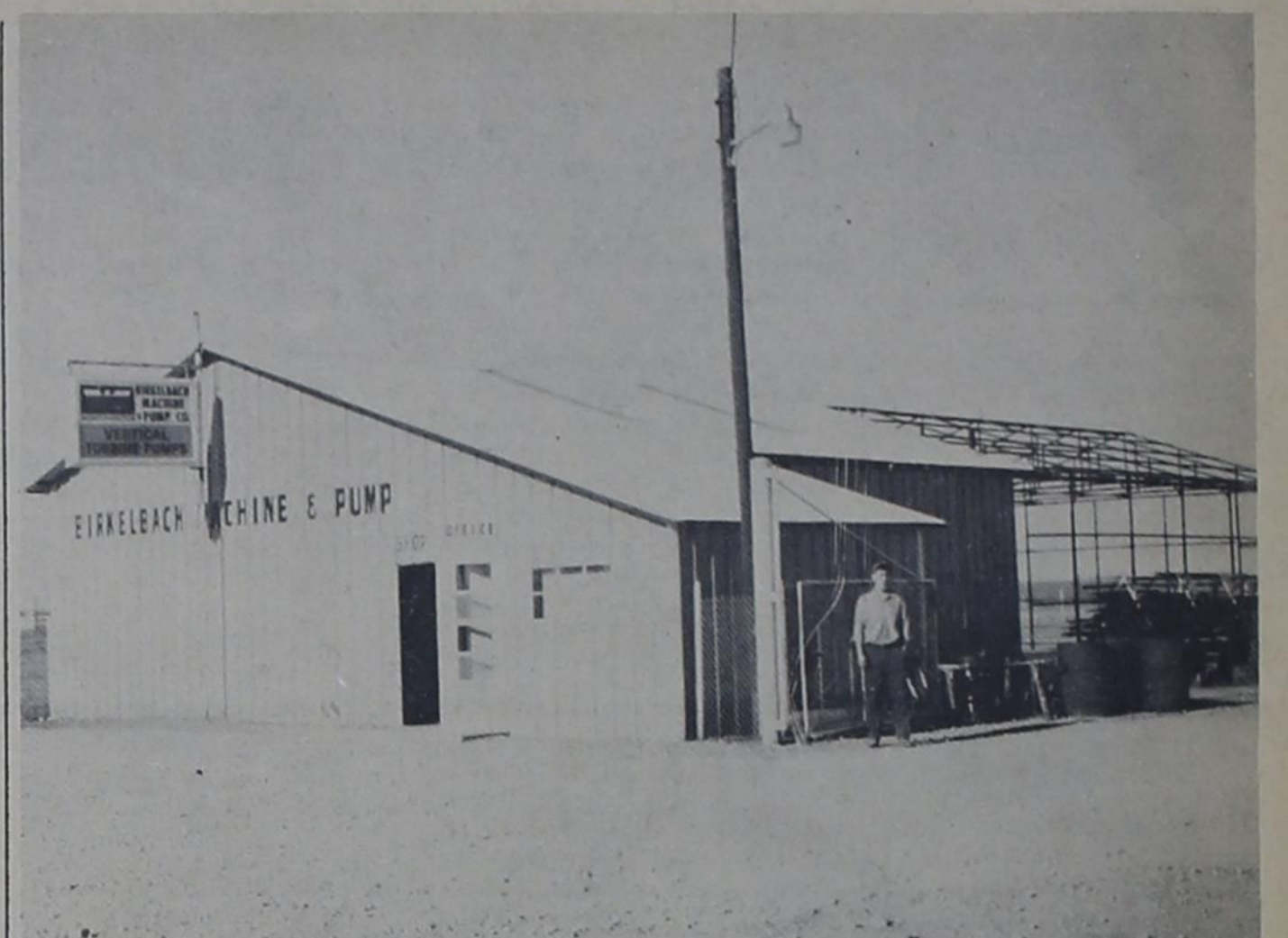
ADDITION -- Birkelback Machine and Pump Co. will double the size of its building when a 30X42 addition is completed at the rear of the present facilities on Highway 86, Kenny Birkelbach said the addition will be used for welding and the front for machinery. The company has been in business here nearly three years.
