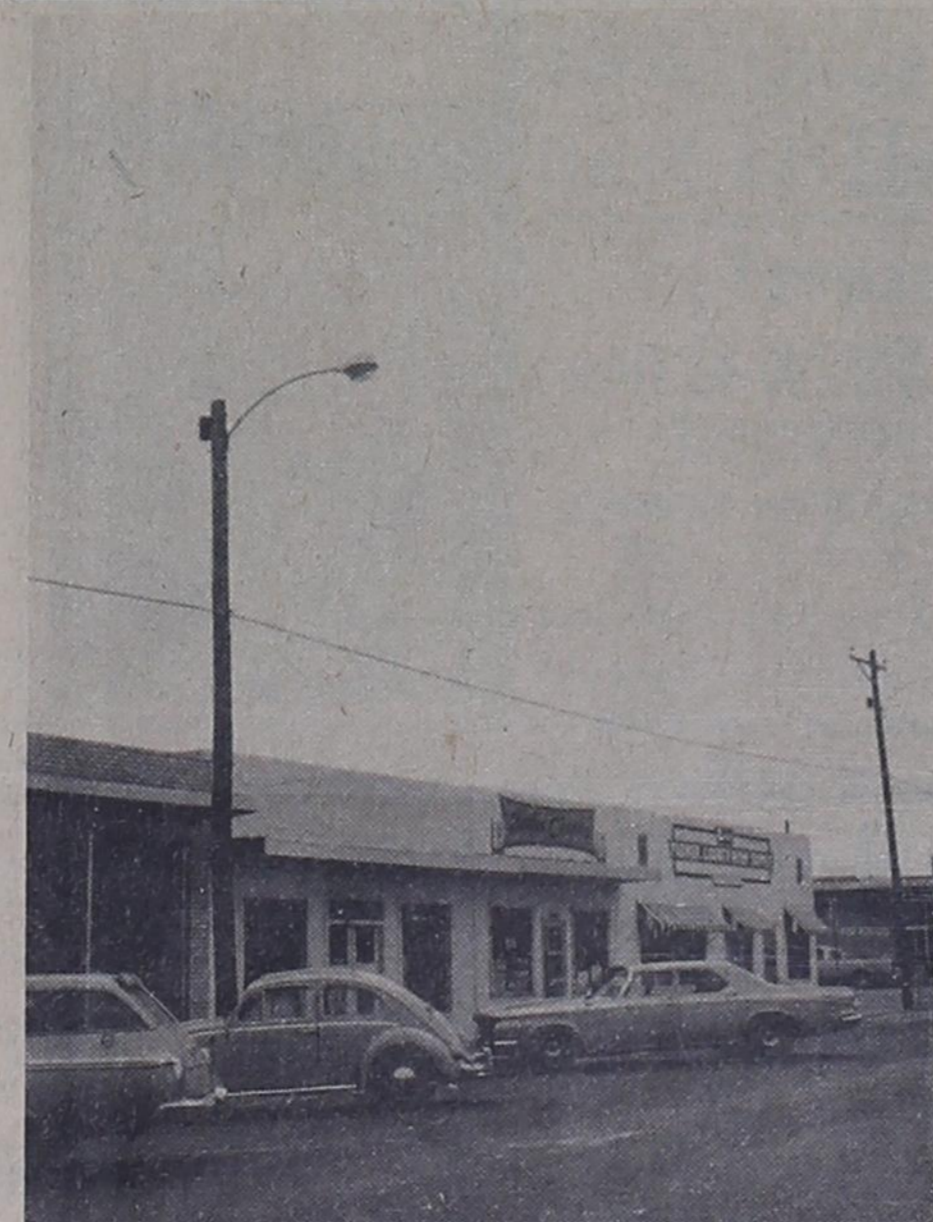
AFTER -- When Southwestern Public Service Company completed its job of removing unnecessary lines and transformers from Main Street in Bovina, only one line was left to service the street lights. Poles were shortened giving the downtown area a neater appearance.
