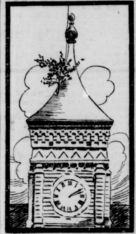
Tree Growing on a Tower.
