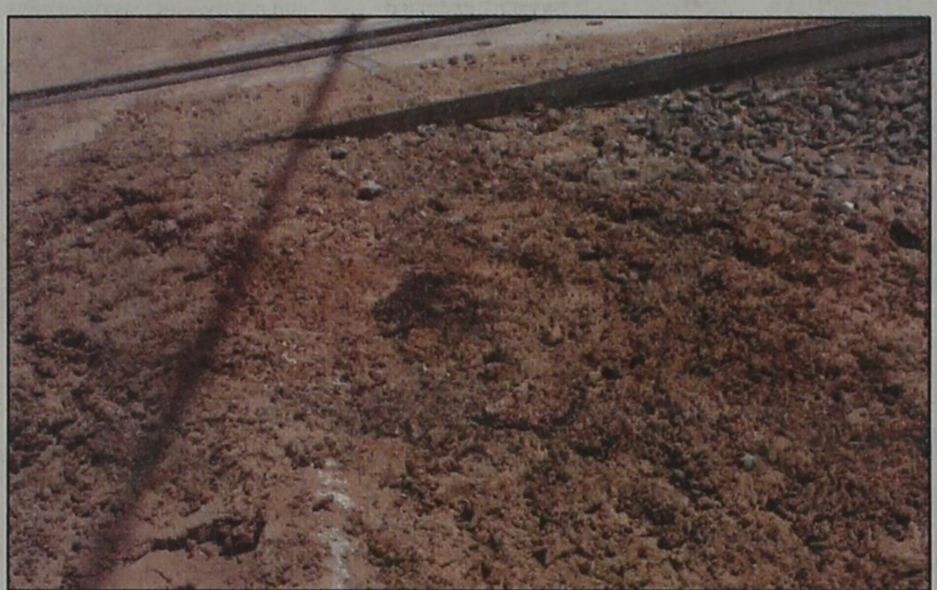
Repaired water main break at 15th and the railroad tracks
