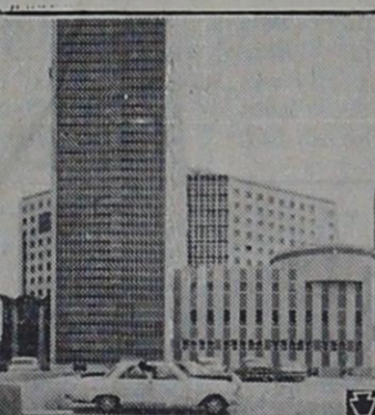
STRIKING design of St. Joseph's Hospital, Chicago, uses Indiana limestone to full advantage. Not only does the famous building stone provide a durable, maintenance-free covering for the building, but it highlights the architect's use of other building materials, with outstanding economy.
