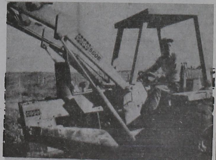
JIM MASON, backhoe operator, building a tank pad on the Edwin L. Cox lease
