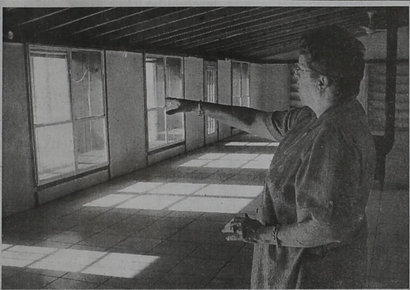
Kenda Bartlett describes the study room inside the CCC Boys' Ranch located west of Post on CR 125. The thick adobe brick walls absorb the heat during the summer season, while the sun rays and wood stove (back) provide warmth during winter.
