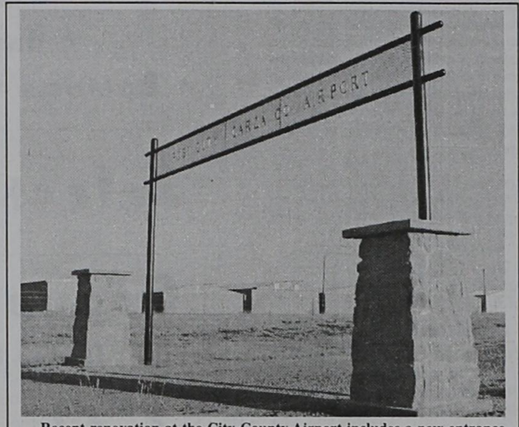
Recent renovation at the City-County Airport includes a new entrance sign. (Photo by Tim Burnett)
