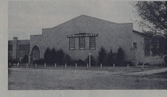
Oklahoma Lane Methodist Church
