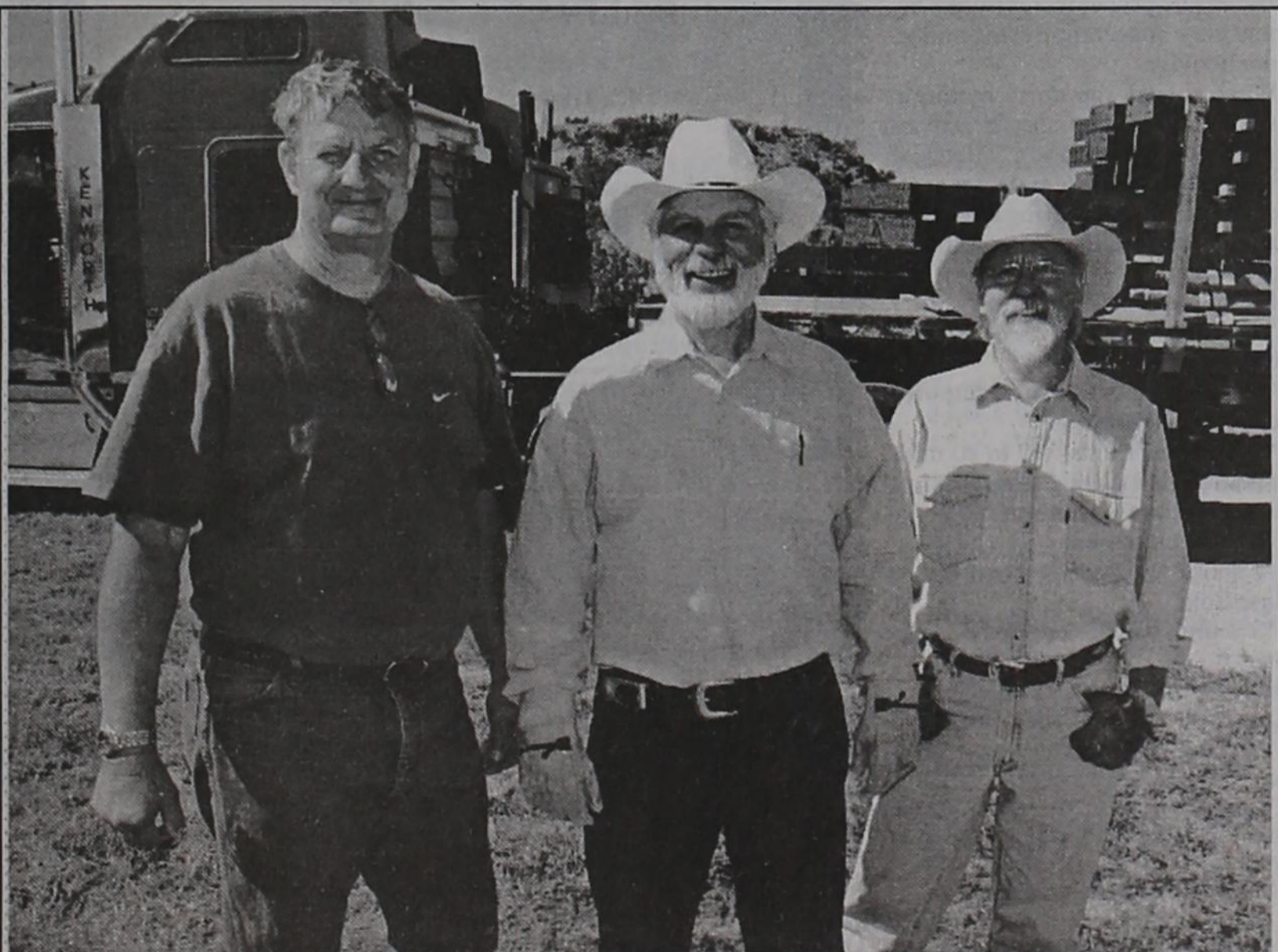
Construction began last week at the "Ragtown" entertainment site located on the grounds of the old Caprock Golf Course. Shown (left to right) Bill Crites, Glen Polk and Chip Polk worked through the day unloading steel beams. (Staff photo by Tim Burnett)
