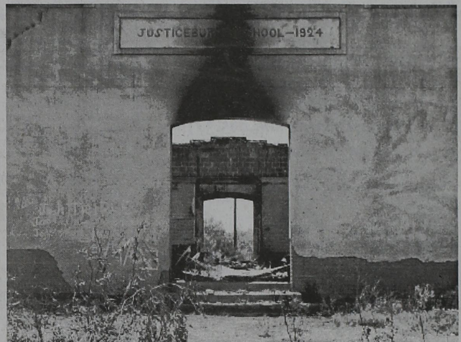
Fire guts historic Justiceburg school building
