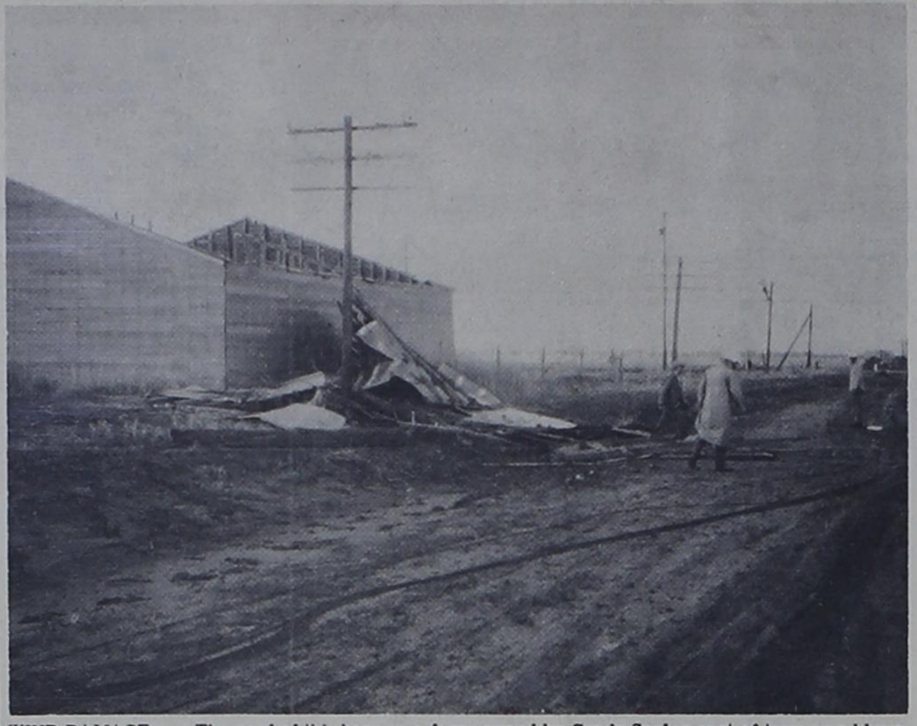
WIND DAMAGE --- The roof of this barn on a farm owned by Grady Sorley east of town was blown into the nearby telephone lines by Friday afternoon's exceptionally high winds. The phone lines, broken by the flying tin and lumber, were repaired Saturday by a Southwestern Bell crew from Amarillo.
