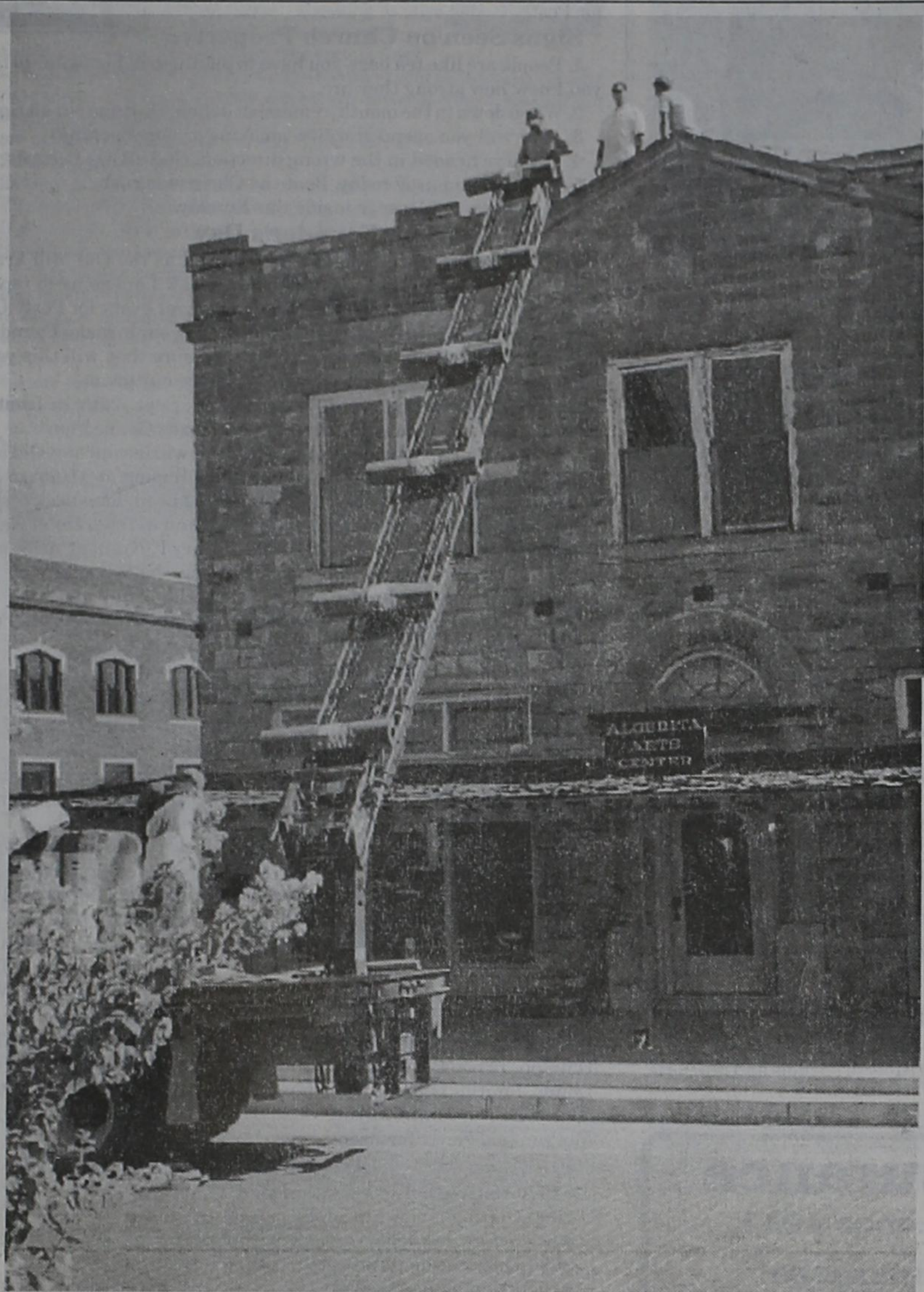
New Roof at Algerita
