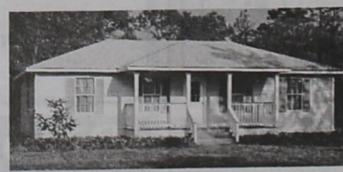
The Arlington, just one of more than 30 home designs you can choose to build on your property.
