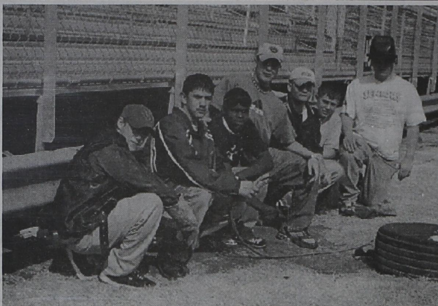
A safety rail has been installed at the PHS football stadium thanks to the efforts of Post High School ag metal fab students. Helping with the project are (left to right) Kurt Moore, Steve Martinez, Gene Bell, Ross Babb, Randy Moore, John Eilenberger and Brian Ellison. Students worked under the supervision of Ag Science teacher Perry Smith.
