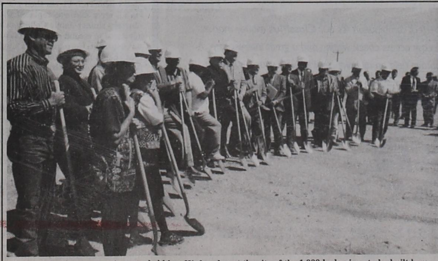
Groundbreaking ceremonies were held last Wednesday at the site of the 1,000 bed prison to be built here. (Photo by Sheri Lewis)
